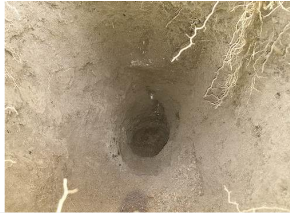
PH3. Footing Probe Test Pit TP1
