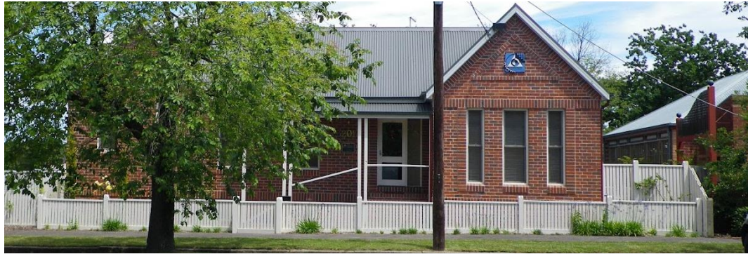
PH1. View over the property from the front
