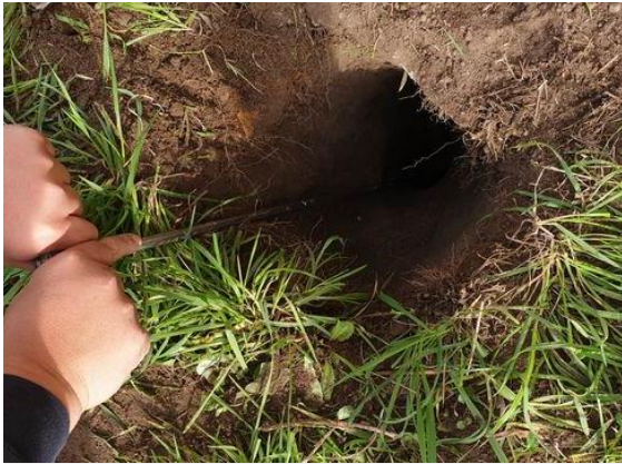
PH2. Footing Probe Test Pit TP1
